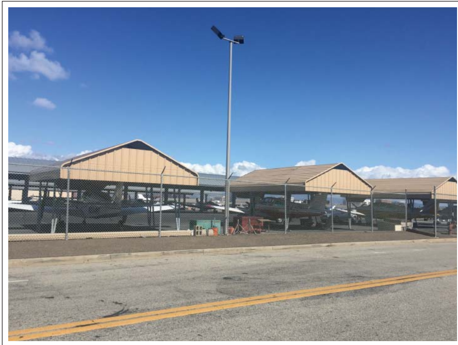
Photograph C: View from Ike Jones Road, east of Airway Avenue, looking north.
