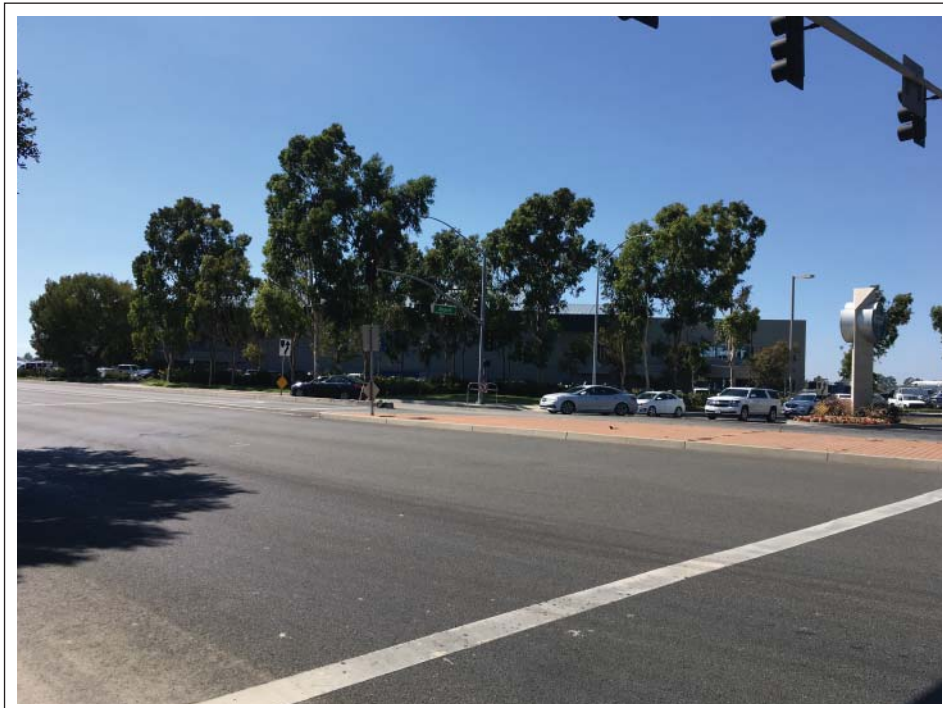
Photograph J: View of the existing Full Service Northeast FBO from Campus Drive.
